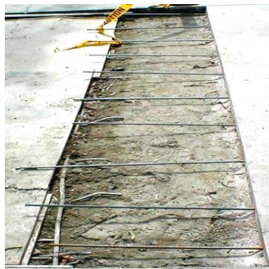
Figure (2-a): Walkway area during the repair process
